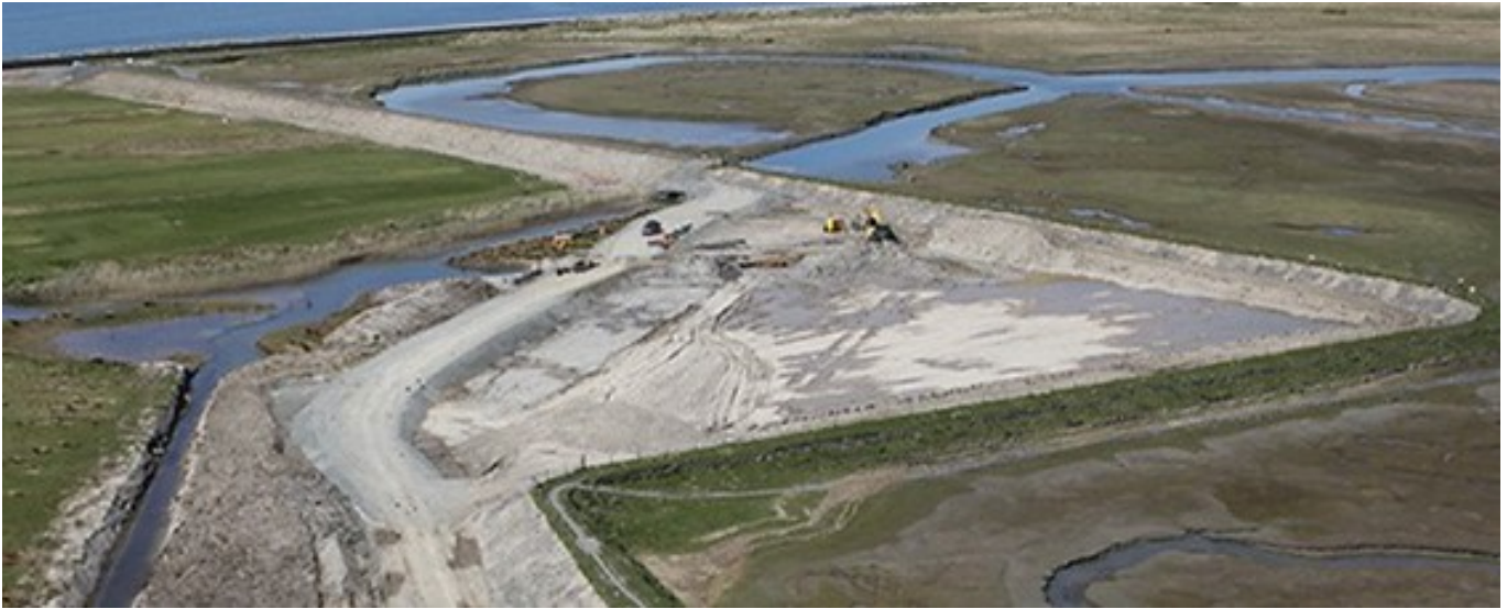
Figure 71: Construction of the Afon Henddol tidal gate, showing the water collection channel.
