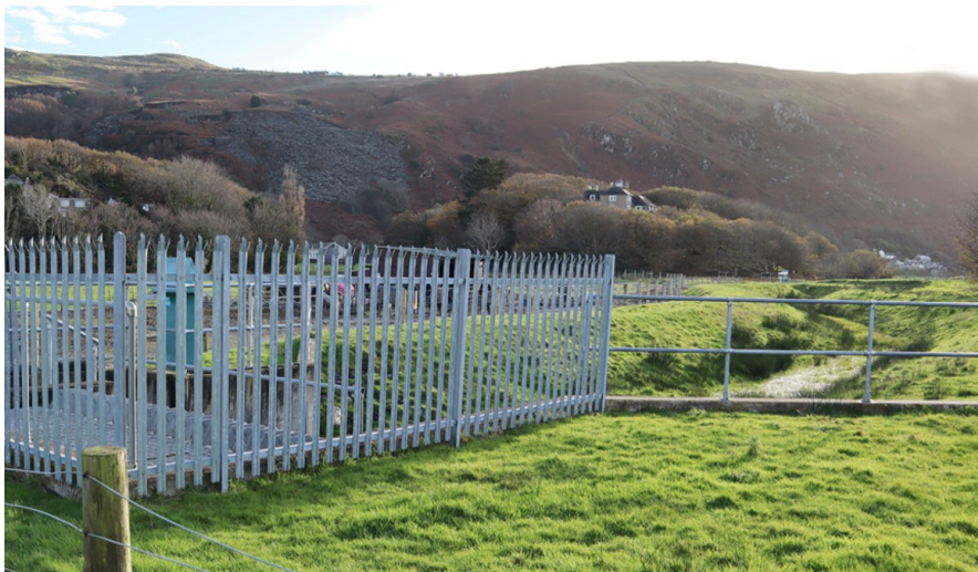
Figure 21 Afon Henddol flood alleviation channel. The structure in the left foreground is the entrance to a culvert beneath the main road at Fairbourne level crossing. This inlet is fitted with a screen to catch flood debris and prevent blockage of the culvert.
