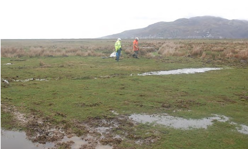
Figure 60 Soil sampling pit excavated close to the line of the proposed new flood embankment (Owen, 2010).
