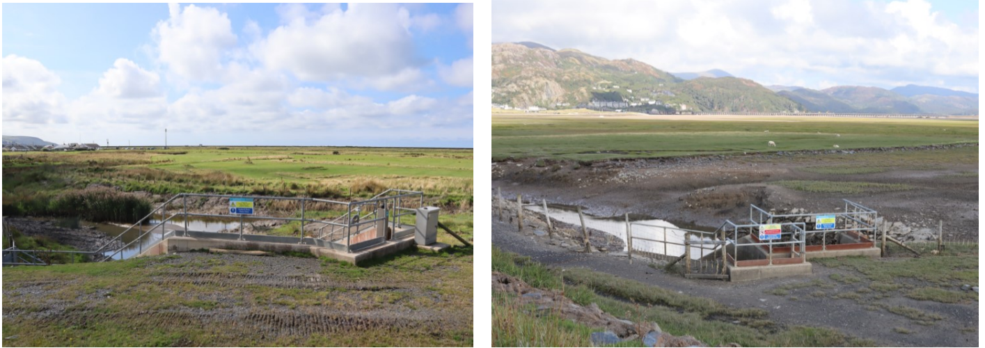
Figure 38: Tidal gate alongside Fairbourne golf club at the mouth of the drainage ditch network. (left) Inlet from the stream channel (right) outlet to the estuary.
