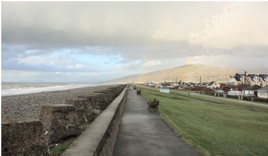
Figure 86: View along the Ro Wen spit, Fairbourne showing the considerable width of the storm beach and landward embankment.
