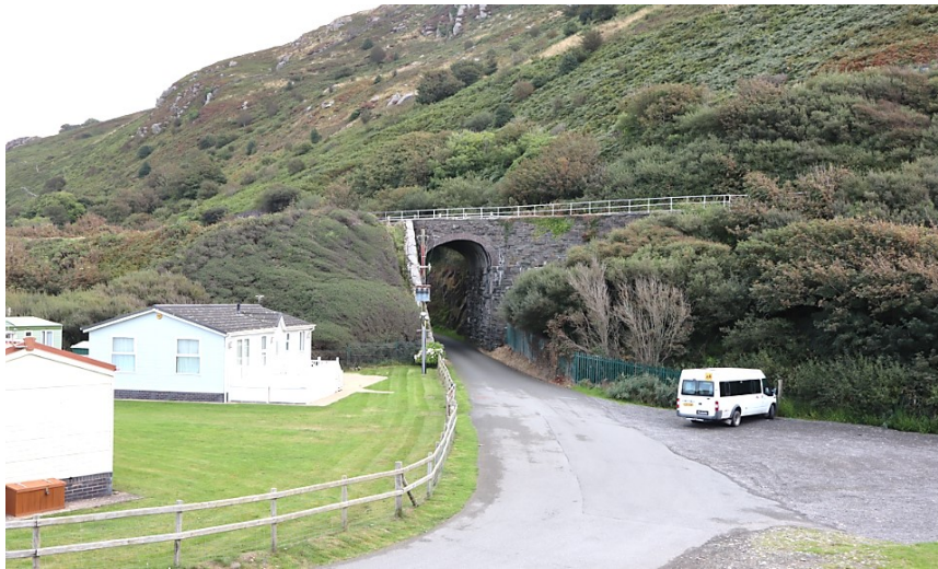
Figure 20 Railway bridge at Friog.
